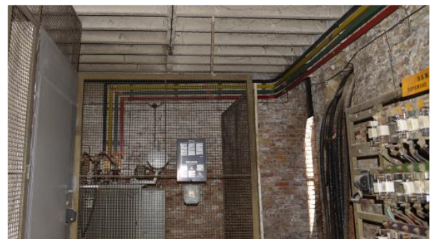
Figure 1. Transformer station in the basement of a residential building (10/0,4 kV, 1 × 1000 kVA) [10]
